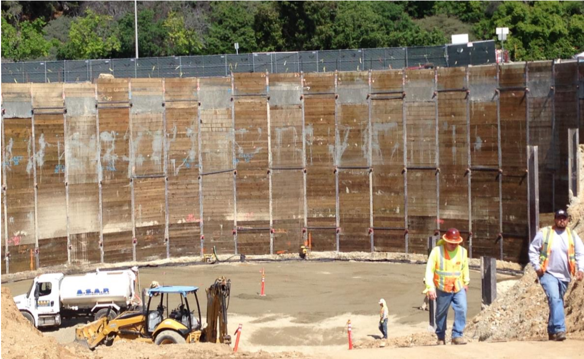
Thermal Energy Storage Tank Construction
