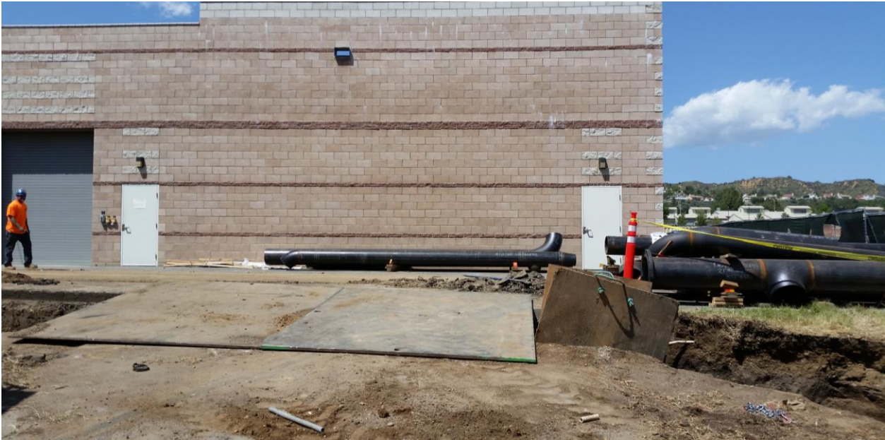
Chiller Cooler Tank Upgrades
